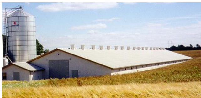
Figure 1. A photo of housing using mixing ventilation with wall jet inlets.
