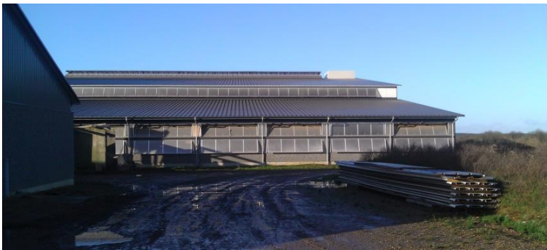
Figure 7. A photo of the dairy cattle building with hybrid ventilation.
