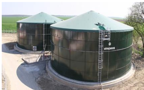
Figure 1. Closed steel manure tanks.
